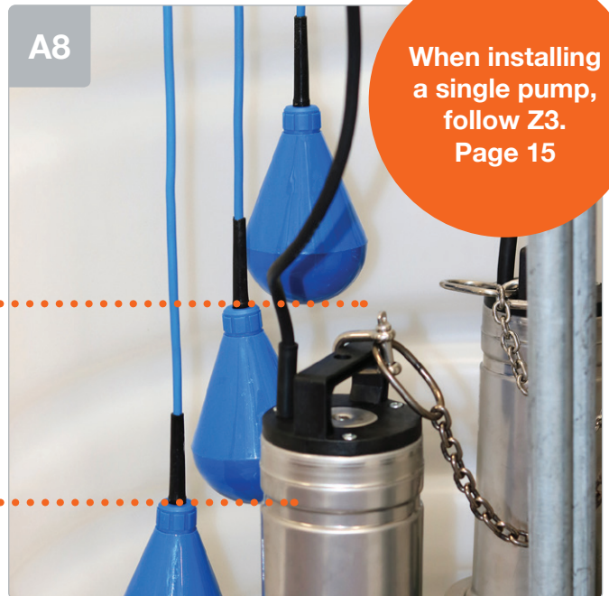
Setup the other two floats so they are staggered with each other. Use the top of the last float for guidance on the height of the next. Be aware that float positions are subject to the incoming inlets and care should be taken to set up the floats correctly with that in mind.
