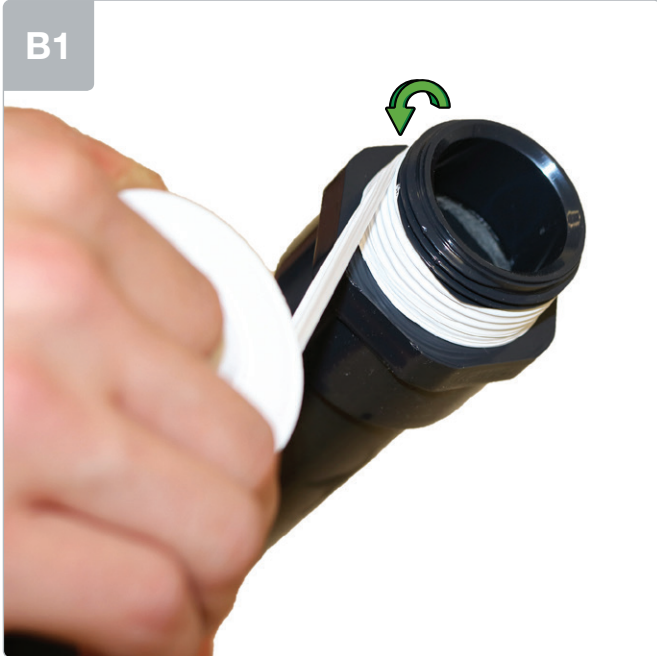
Wrap the thread of each male iron on the end of the discharge pipes with PTFE tape.
